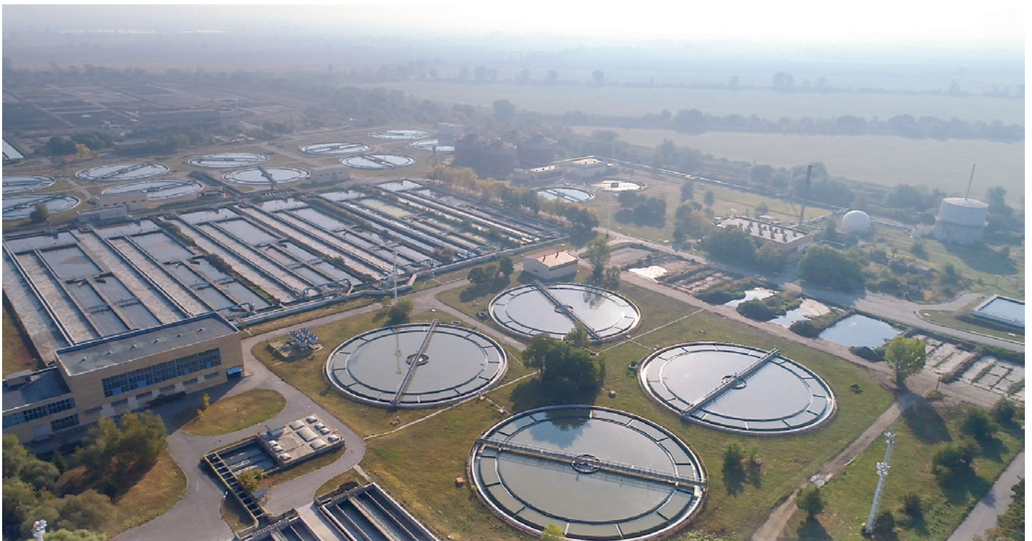
Wastewater treatment plants are strategic assets to produce biogas and biomethane for local needs, across Europe. Here the Kubratovo wastewater treatment plant operated by Veolia on behalf of the City of Sofia (Bulgaria)
