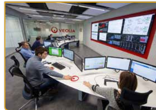
In December 2015, Veolia inaugurated its Hubgrade in Bilbao, Spain. This platform oversees, remotely and in real time, over 2,000 of the Group’s energy facilities across Spain. It collects and analyses data, set the interventions of Veolia technicians in motion on customer sites, and as a result help achieve up to 15% additional energy savings.
