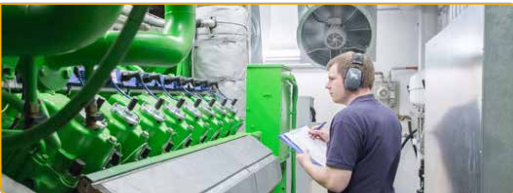
In Braunschweig, Germany, Veolia converted fossil fuel powered central heating installations into a biomass cogeneration plant and a wood boiler. Two thermal storage units with innovative insulation also help ensure low heat losses. In total, the new installation provides 8,000 T of CO 2 savings annually. It relies on locally available waste wood supplies.
